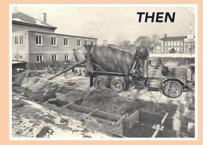
**In 1978** - Falmouth Ready Mix, a local producer, supplied the concrete for the east wing of the Falmouth Public Library. On this cold April day, concrete mixers line up to begin pouring the huge footings that will support the walls of the east wing addition. Concrete technology, placement and the industry as a whole have gone through many changes since then.
